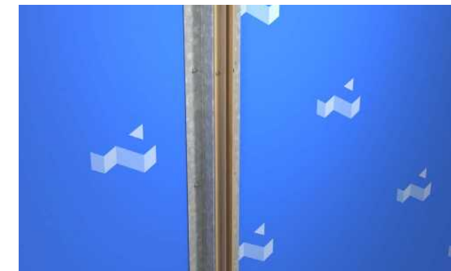
Step 1. Screw the C Joiner Trim to the centre of the top hat or structure.
